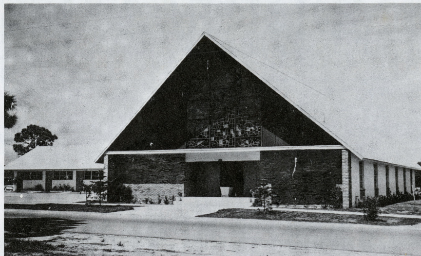
One of the first of the 32 churches built over the past five years in South Atlantic Conference is located at Fort Lauderdale, Florida. The building is air conditioned with a seating capacity to accommodate 500 members. The property is valued at $125,000 and the pastor is J. P. Monk.
