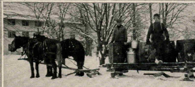
WATER SUPPLY FROM LEMON CREEK.
